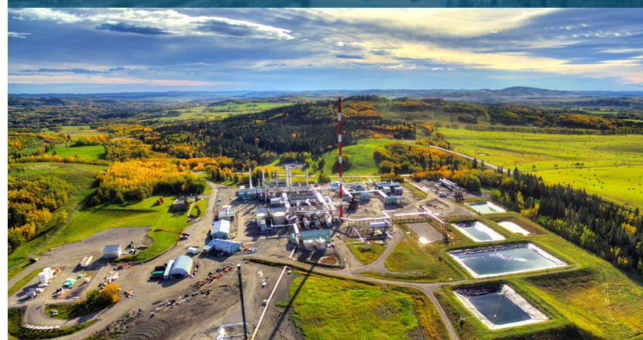
Quirk Creek Processing Facility
